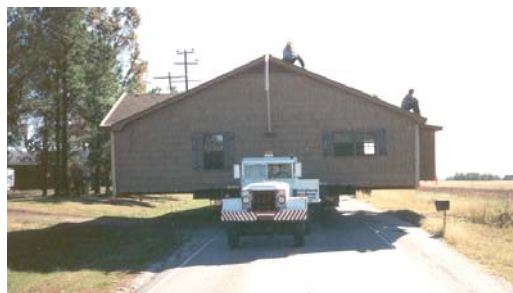
Small, wood frame buildings are the easiest to relocate
